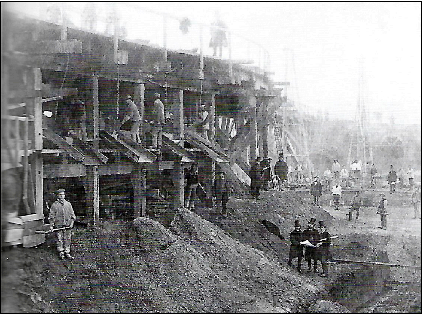
Building the Northern Outfall sewer, 1862
